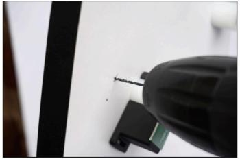
And fix the reader with the screw - do not tighten it yet:
