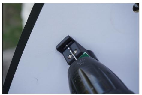
Fix the reader to the side wall making sure the housing does not move. You can always loosen the screw to adjust the position of the reader.
